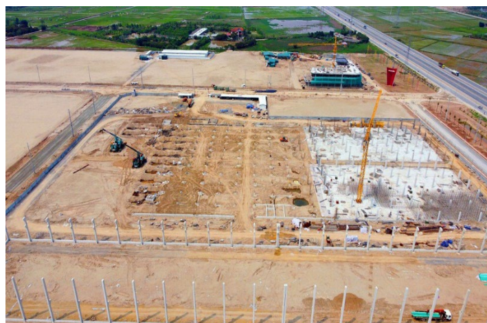
Figure 2: Current status of the Dang Le Industrial Cluster (part of the Hung Yen Industrial Cluster) – land leveling completed, and factory construction is underway.
