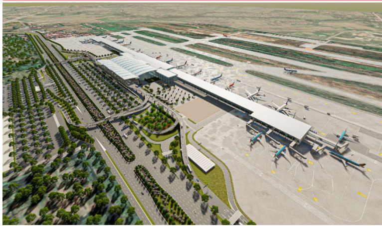
Figure 31: Expansion of Terminal T2 – Noi Bai
